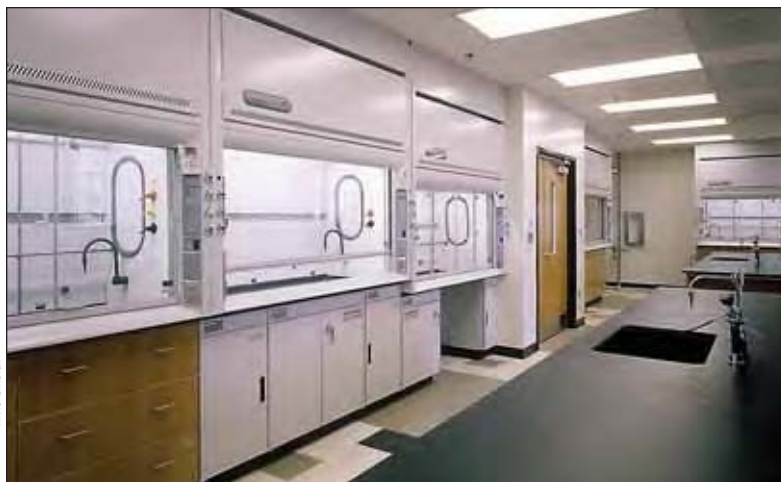
At Meredith College, Raleigh, North Carolina, Protector XL Laboratory Hoods mounted on Protector Acid and Solvent Laboratory Hoods alternate with Protector XL Laboratory Hoods mounted on wood casework. One hood is mounted lower and with accessibility underneath for a wheelchair.
