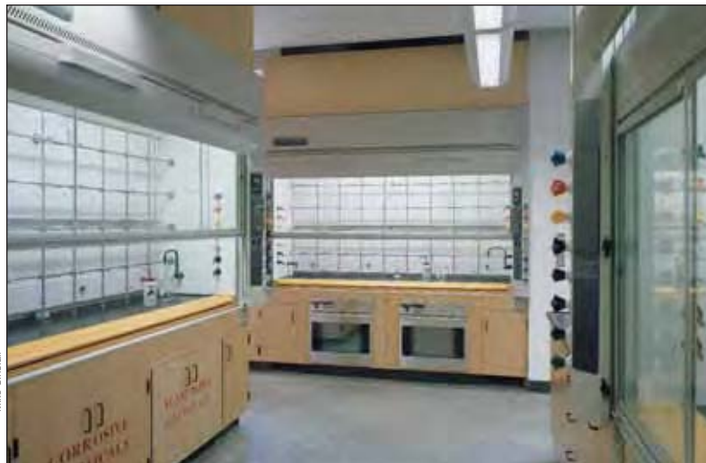
At the University of California-Riverside, each Protector XL Laboratory Hood is outfitted with sixteen service fixtures, including gooseneck faucet and turret. Distillation grids are mounted to the hood walls to provide ample areas for suspending apparatus and glassware.
