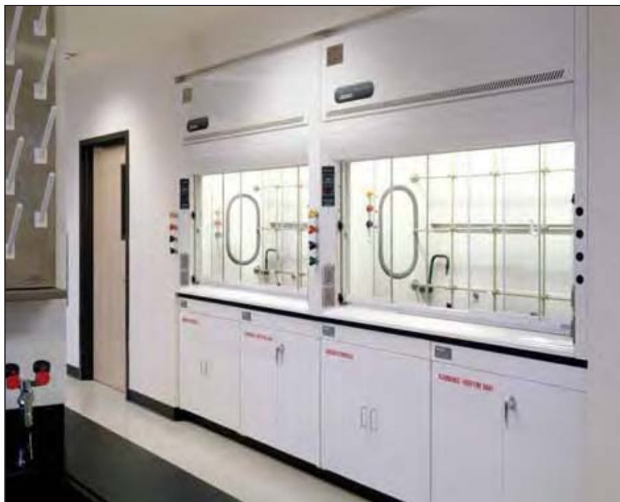
The Protector XL Benchtop Laboratory Hoods installed in this laboratory feature combination vertical-rising/horizontal-sliding sashes.
