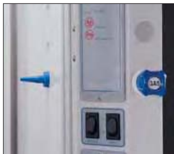
Color-coded fixtures provide at-a-glance service type identification.
